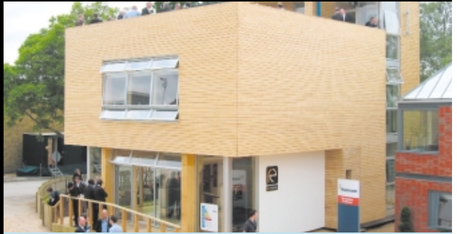
● IMAGE: The Re-Thinking school has raised the bar with its sustainable offsite building approach.
